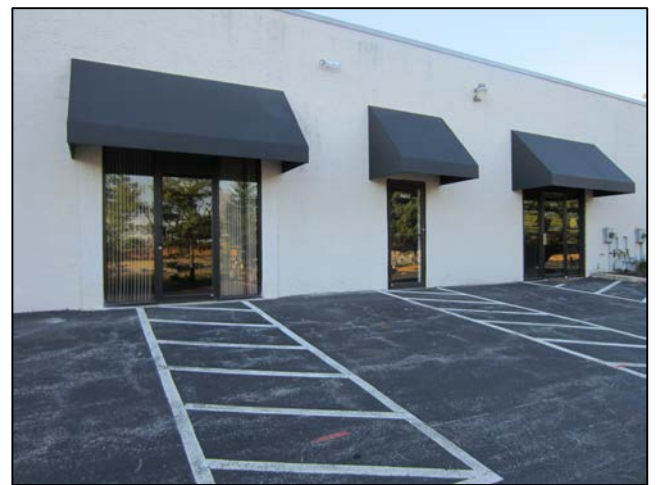
Rear Office Entrance
