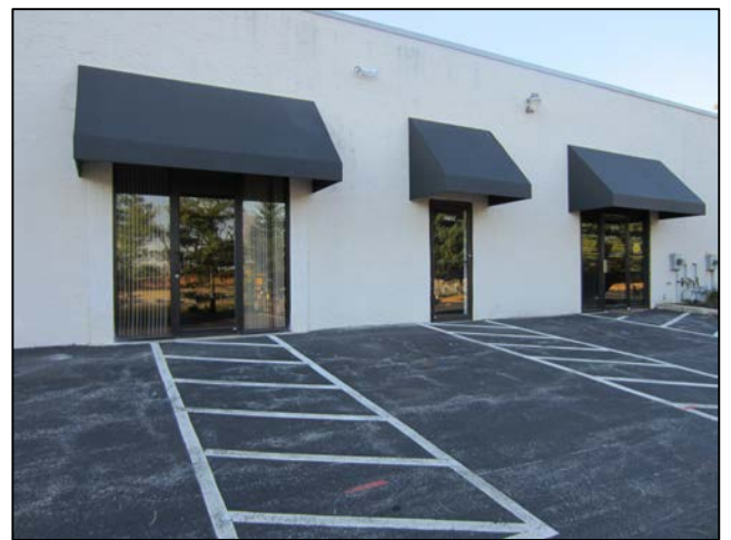
Rear Office Entrance
