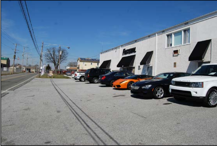
427-431 South Bolmar Street
